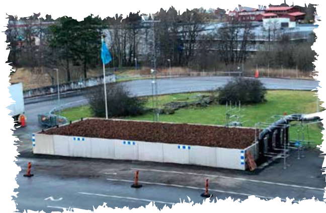
Biobed at our factory in Kungälv, Sweden.
